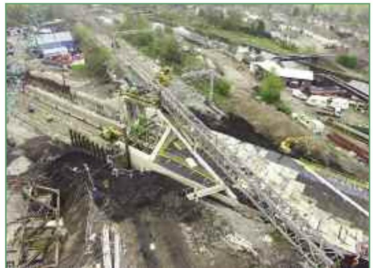
The award-winning box-jacking at Tipton in the West Midlands to remove the last level crossing on the west coast main line. (Top) Preparing the box and jacking equipment. (Above left) Part way through the jack. (Above right) Jack completed and preparation under way for reinstating the track.
