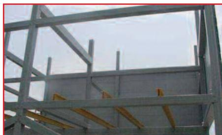
Cooling tower structure of pultruded FRP shapes
