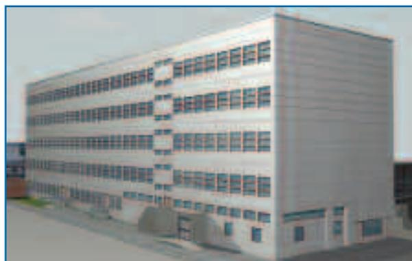
Over-clad building using 'rain screen' metallic cladding.
