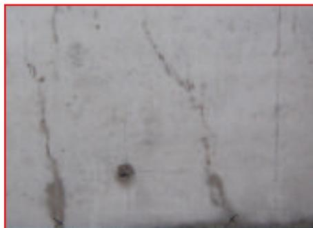
Early-age thermal cracking in a wall on a stiff foundation
