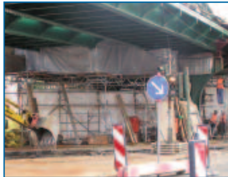
Road and rail construction work
