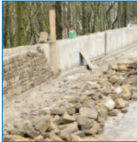
Rebuilding of a drystone wall
