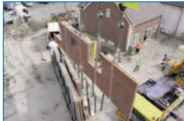
(Above left) One of the prefabricated cavity wall panels being craned into position
