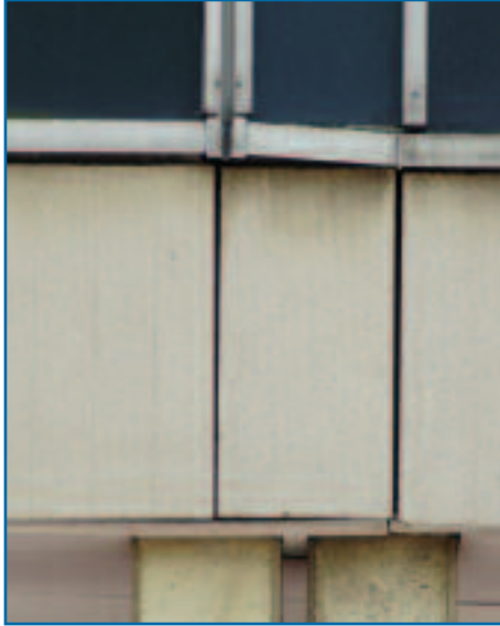
Cladding bridged across separate structures
