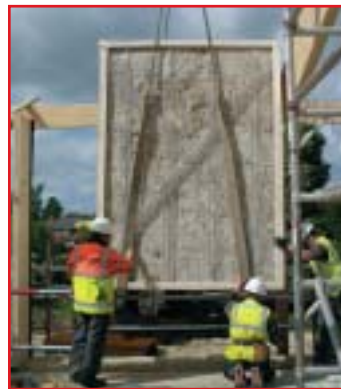
(Left) York EcoDepot, clad in ModCell panels (Right) Installation of ModCell panel at York EcoDepot
