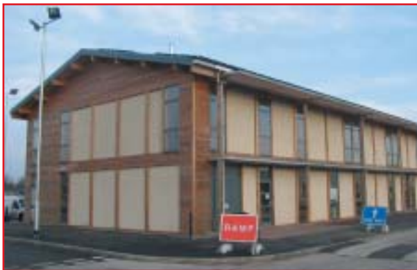
(Left) York EcoDepot, clad in ModCell panels (Right) Installation of ModCell panel at York EcoDepot
