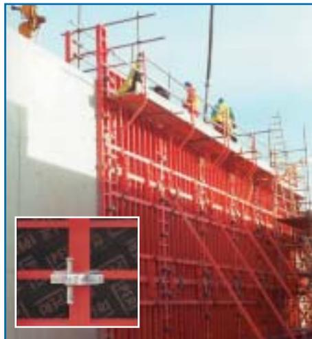
Standardised panels with integrated walkway system (Inset) Innovative coupler design allows rapid panel joints (both courtesy Peri Ltd).
