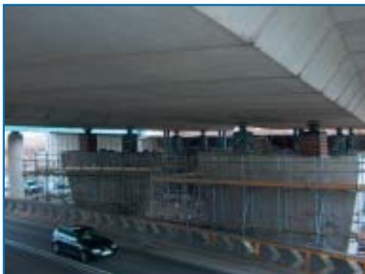
Temporary jacking at Princess Parkway prior to installation of permanent steel support columns
