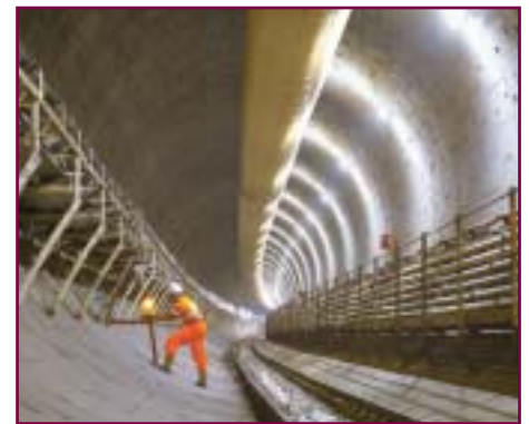
CTRL: Tunnel 250: May 2002 QA Photos Ltd: courtesy of Rail Link Engineering
