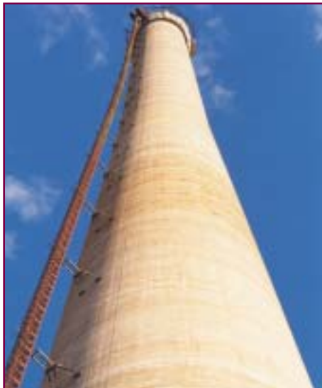
(Top) Quick and efficient construction with pre-cast elements (Courtesy of The Concrete Society) (Above) In-situ slipformed concrete tower; an alternative to the precast option (Courtesy of Bierrum)
