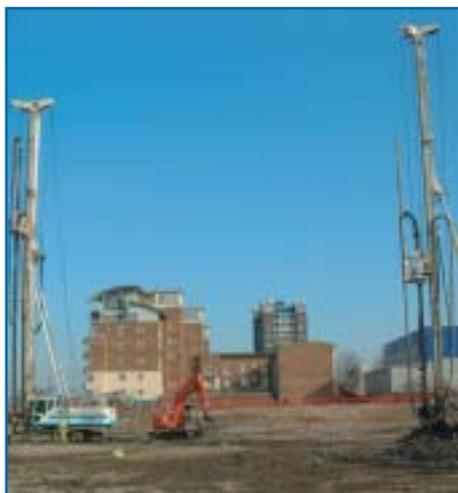
*Piling at urban, brownfield sites can produce large amounts of spoil, which is sometimes contaminated. Displacement augered piles avoid this and can offer economies in design through improvement of the soil*
