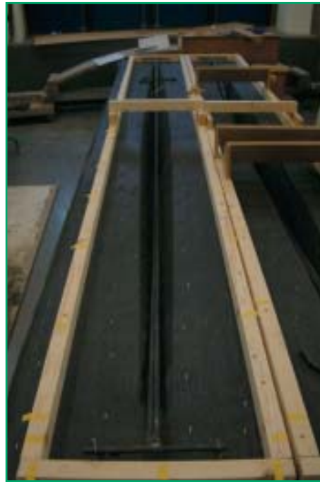
(Above) Example of fabric formwork for a concrete beam.
