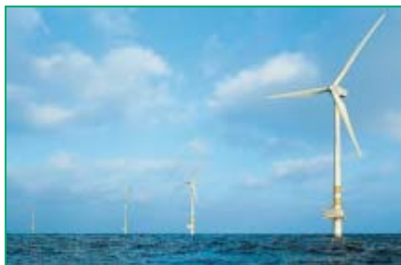
Offshore wind turbine (photo: GE Wind Energy)
