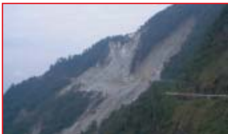
(Top) Developing GIS models and training of staff from the Bhutan Department of Roads (Above) Road blockage and loss of carriage-way at Jumbla on the Phuentsoling-Thimphu Highway, Bhutan
