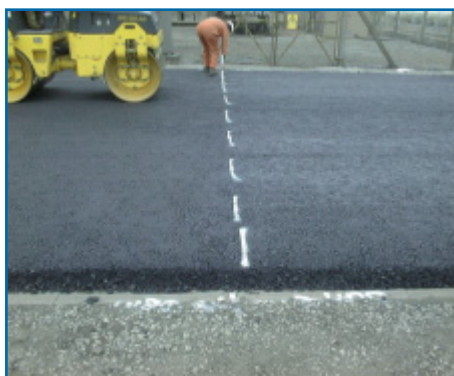
The demonstration road, the right-hand side of which contains the ISF slag, the left-hand side the control mix.
