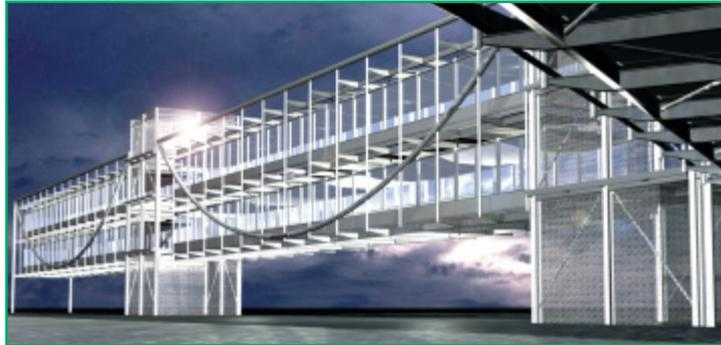
*Pier 3 at Gatwick. It is an impression of the Pier Segregation project that will start on site this December and utilises BAA's off-site manufactured corridor*
