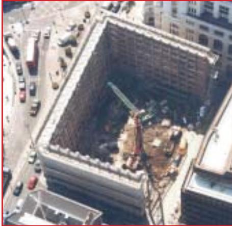
façades retained using different systems and configurations on projects of different sizes and complexity. A step-by-step calculation for the wind loads on a façade using BS 6399-2 and a worked example are included.
