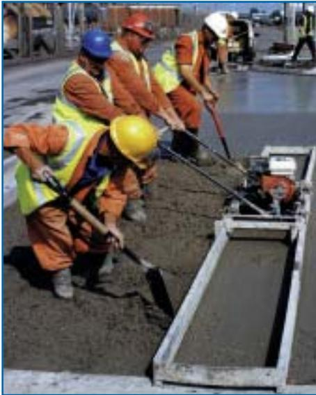
Construction of trial access road using non-ferrous industry waste as aggregate
