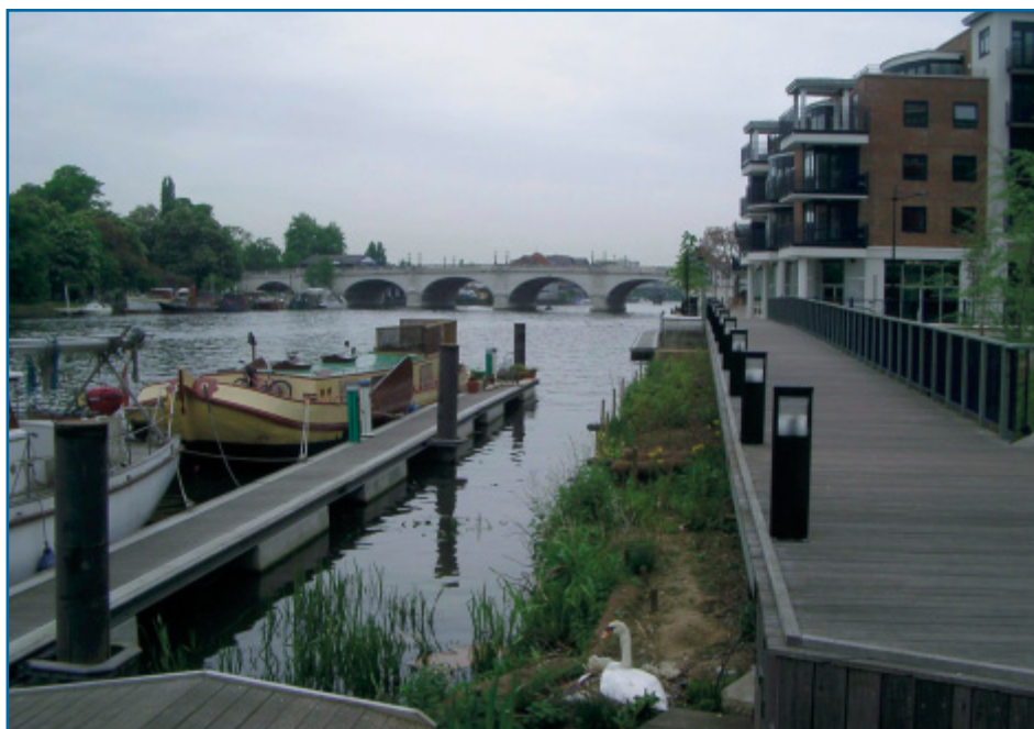
Artificial banks and nesting sites introduced to a new riverside development at Kingston upon Thames (photo courtesy of Crane Environmental Ltd)
