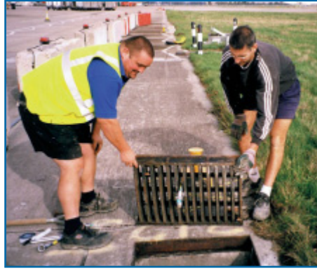
Installing monitoring equipment at Heathrow Airport
