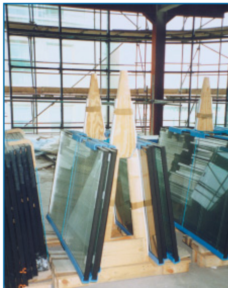
Glazing Units stored carefully on site to avoid damage
