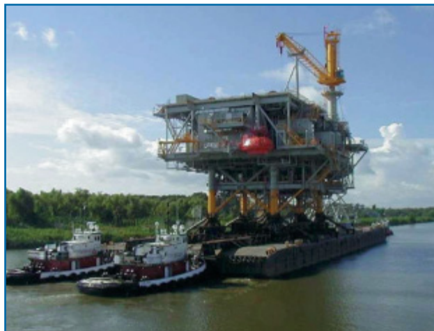
The topsides for the Hibiscus Offshore Platform, Trinidad
