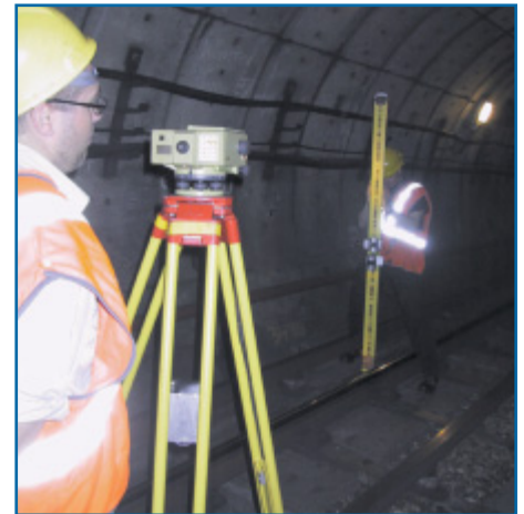
Taking measurements underground
