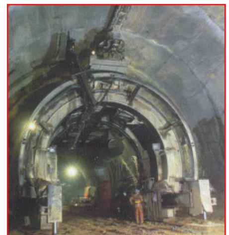
Perforex tunnelling machine
