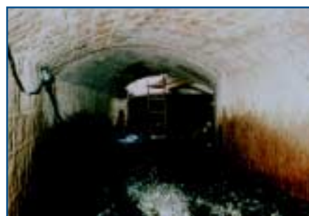
Surface water with culvert
