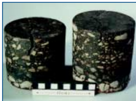
Top-down cracking of hot mix asphalt
