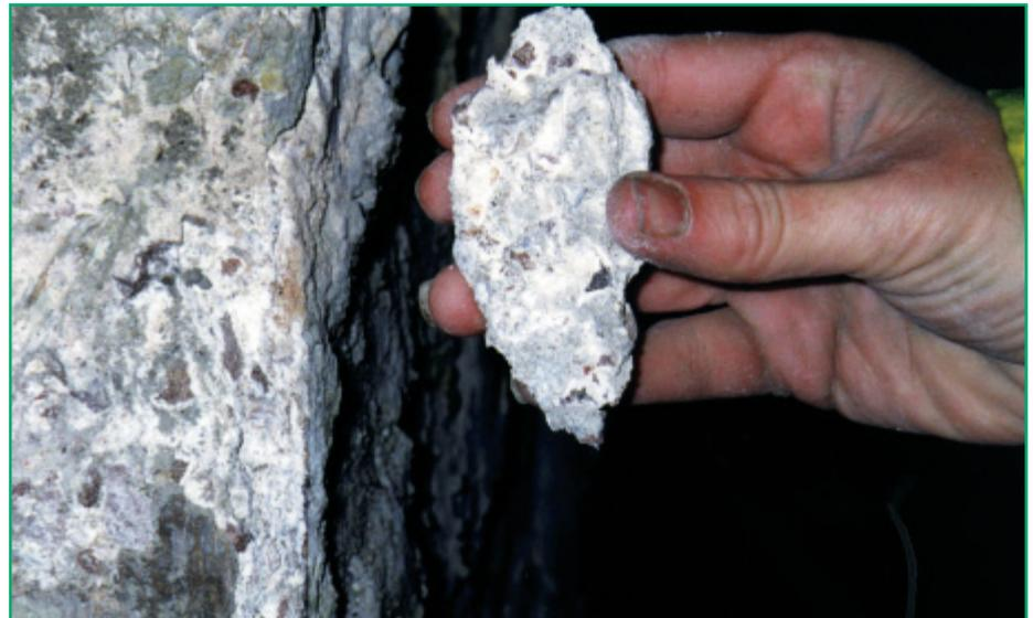
Concrete subjected to the thaumasite form of sulfate attack can become friable enough to be dislodged by hand
