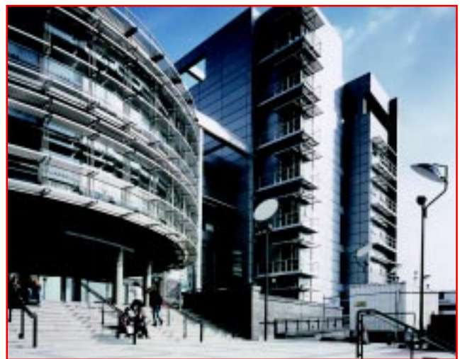
Rainscreen overcladding (Photo courtesy of Allscott Contracts)
