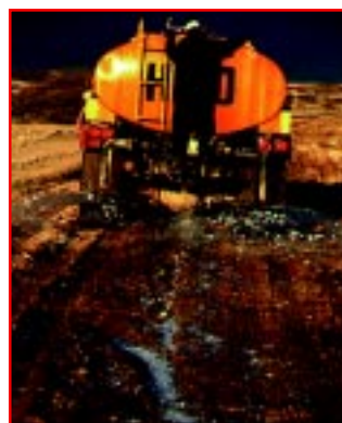
Tanker spreading additives prior to mixing
