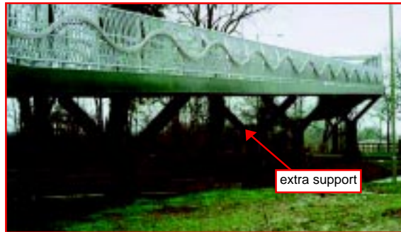
A40 Cutteslowe Bridge showing additional ramp support
