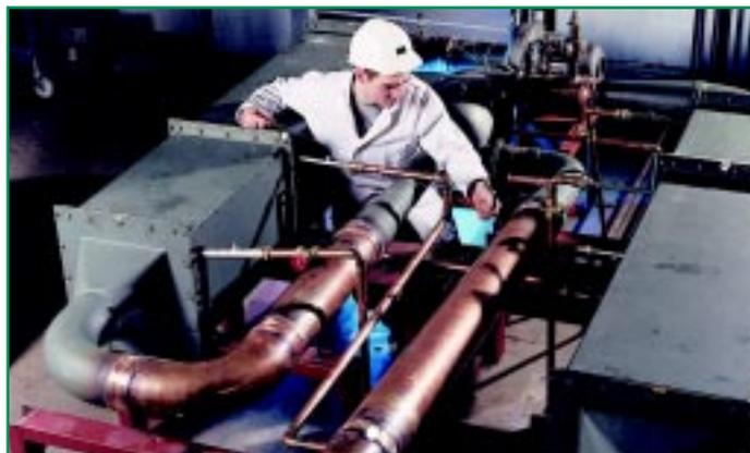
A working demonstration system has been built to heat and cool a suite of offices at the University of Bristol using a standard 4-pipe fan coil system – see accompanying illustration.
