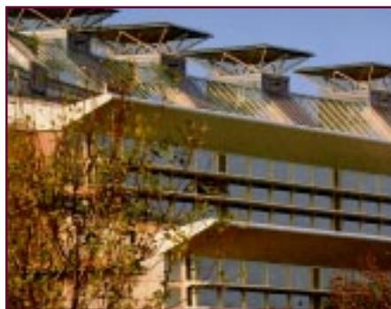
to achieve the air volume flow rate. Adjustments to compensate for factors – including (i) the position and extent of openings, (ii) building resistance and (iii) the height of the wind tower above the roof – are made at this stage.
