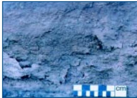
Figure 1: Outer surface of a highly weathered quartz sandstone from a one hundred year old church in East Belfast subject to ongoing high concentrations of atmospheric sulphur, particulates and marine aerosols (photograph, P.A.Warke).
