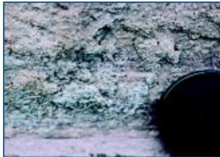
Figure 2: The surface of the same church as in Figure 1, approximately six months after the outer 1 cm of overtly weathered stone had been physically removed. Note the efflorescence formed as the reservoir of salt left in the stone is mobilised and the beginnings of a new cycle of flaking and scaling (photograph, P.A.Warke).
