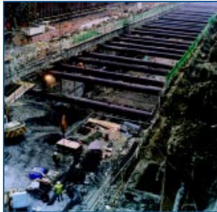
Temporary props in place during construction of Canary Wharf Jubilee Line Extension station (courtesy: Tarmac Construction).
